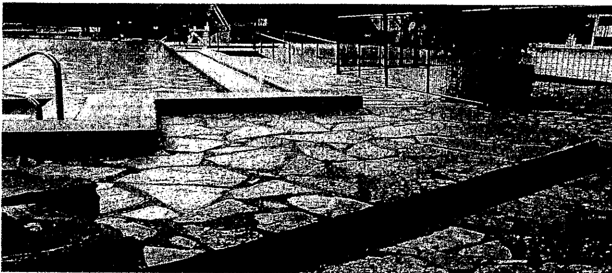
Slipping and tripping hazard
